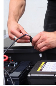
7 3-CORE CONTROL CABLE -> 3-CORE CONTROL CABLE PLUG (LABELLED RW)
